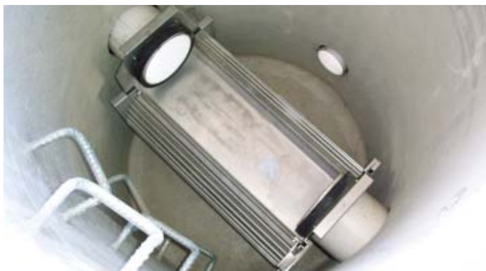
Large-capacity stainless steel filters remove debris and wash it into the stormwater system.
